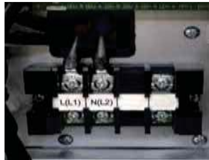
Figure 46: ARUN060GSS4 and ARUB060GSS4 Error No. 22 Compressor Terminal and Wiring Connections.
