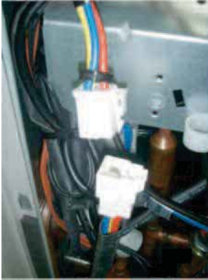
Figure 44: ARUN060GSS4 and ARUB060GSS4 Error No. 21 Compressor Terminal and Wiring Connections.
