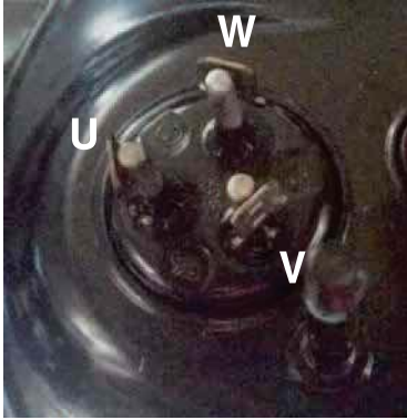
Compressor wiring connections.
