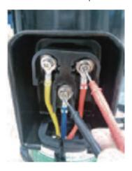
\* Measuring input voltage
