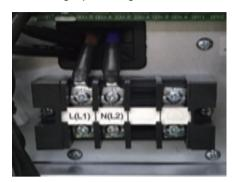
\* Compressor wire connector connection
