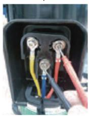
\* Measuring input voltage
