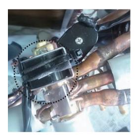
\*\*\*\* Check the output voltage of terminal socket during heating operation
