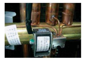
Check the output voltage of the terminal socket during heating operation (output should be 230 V AC).
