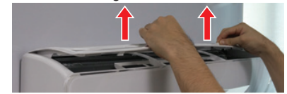
Figure 100: Assembling the Air Filter (Appearances May Vary Depending on Indoor Unit Model).
