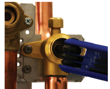
Figure 76: Opening the Service Ports.
