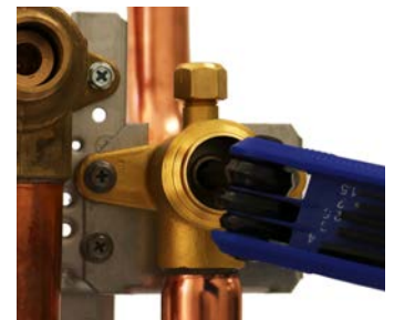
Opening the Service Ports.
